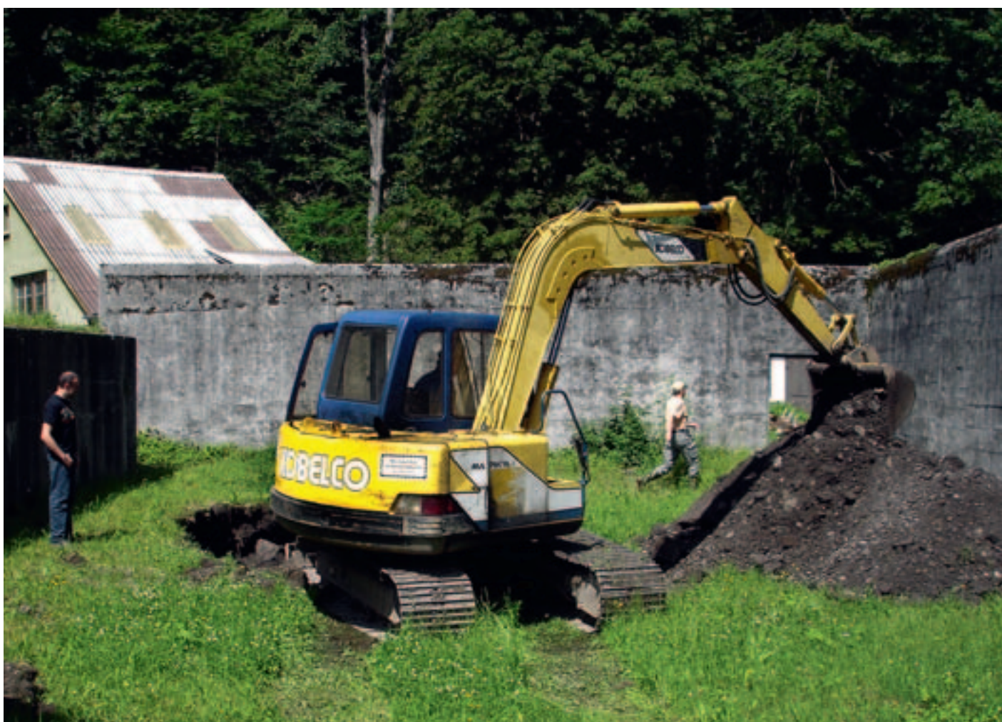
Remediation of a contaminated site formerly used by a Swiss explosives manufacturer: with the aid of isotope analysis, degradation processes in the sub-surface can be reconstructed.
