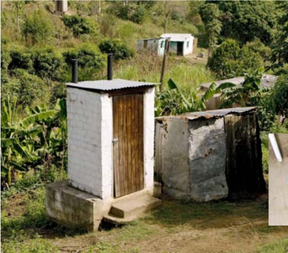
Urine-diverting dry toilet: the innovative technology used for the facilities in Durban (South Africa) is only visible on closer inspection.
