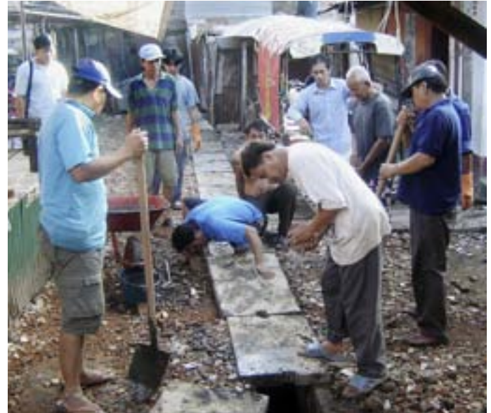
Residents of Hatsady Tai – a low-income district of Vientiane, the capital of Laos – constructing new wastewater infrastructure.
