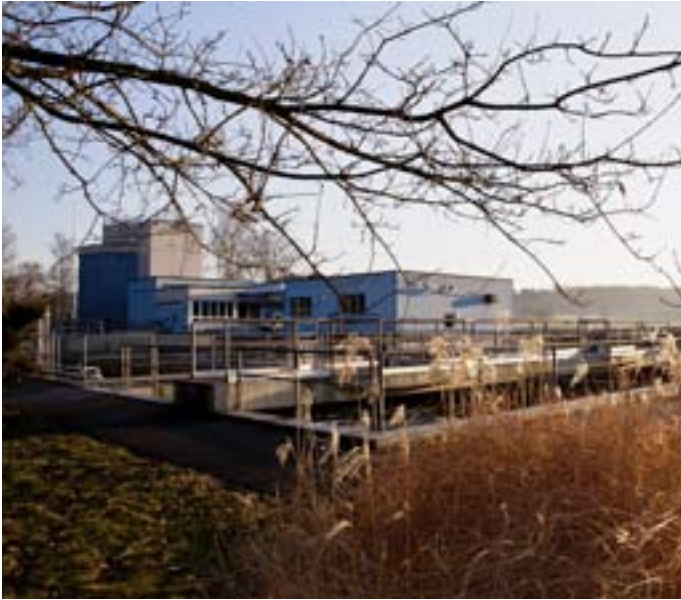
The Mönchaltorf WWTP (Canton Zurich) is one of the plants involved in the SWIP project, which aims to optimize the planning process and develop specific planning measures for the water supply and wastewater management infrastructure of various communes.
