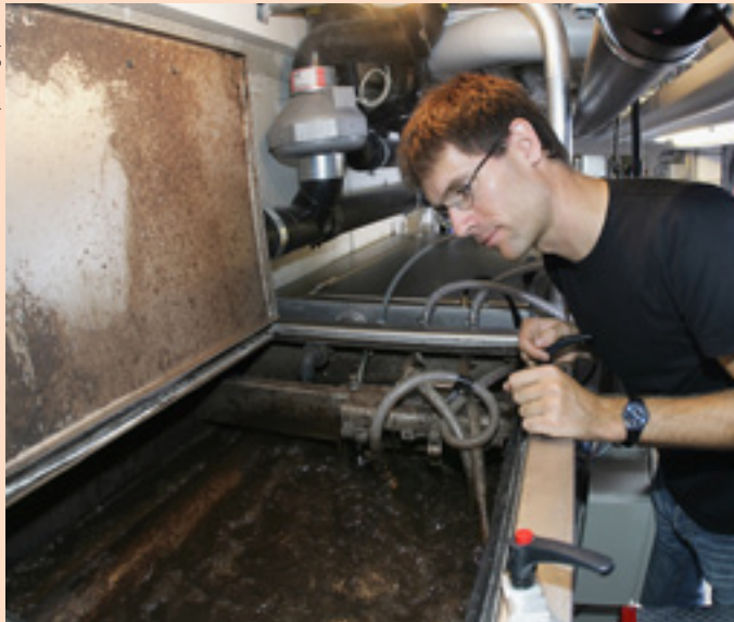
Not to be underestimated: a pilot treatment system in a Swiss household.
