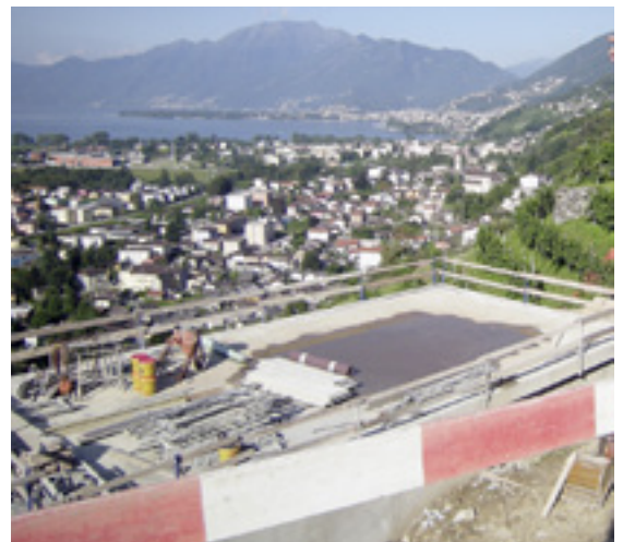
The construction site of the new reservoir, where a drinking water power plant is also being installed.
