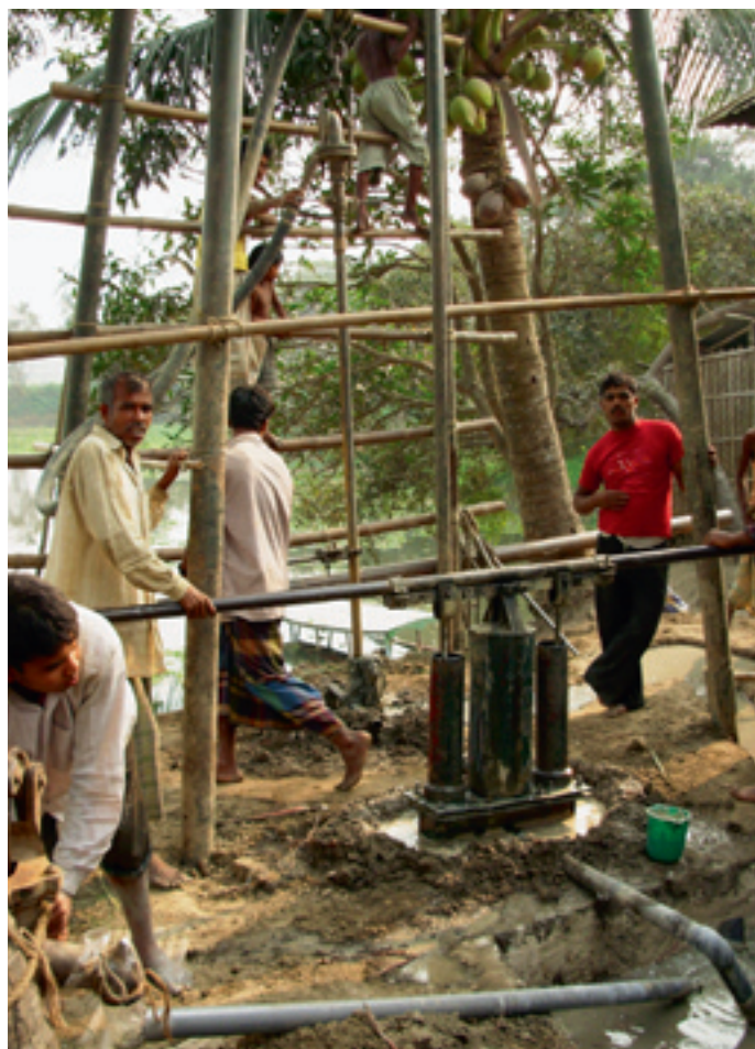
In search of arsenic-free groundwater: a drilling team in Sreenagar (Bangladesh) installs a 220-metre-deep tube well in the soft sediments of the Bengal delta.
