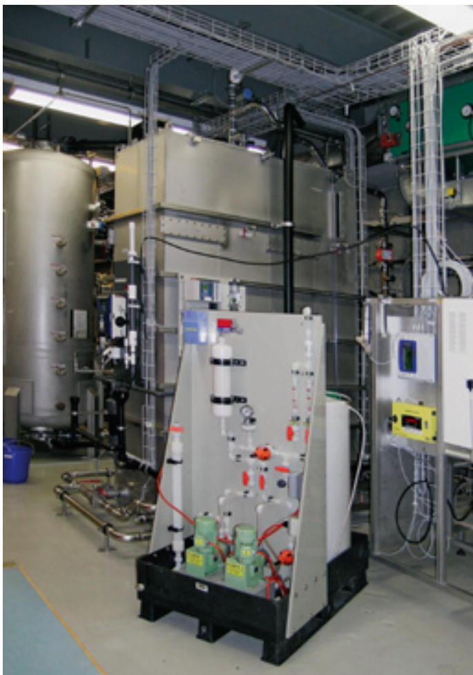
Pilot plant for treatment of Lake Zurich water at the Lengg facility.
