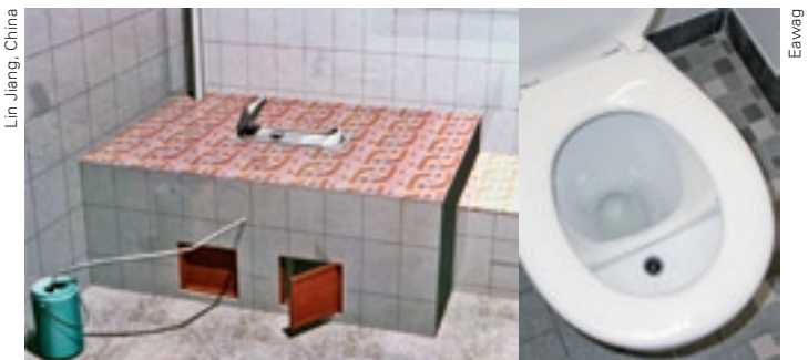
Fig. 2: Two urine-separating sanitary systems: waterless toilet (left) and NoMix flush toilet (right).
