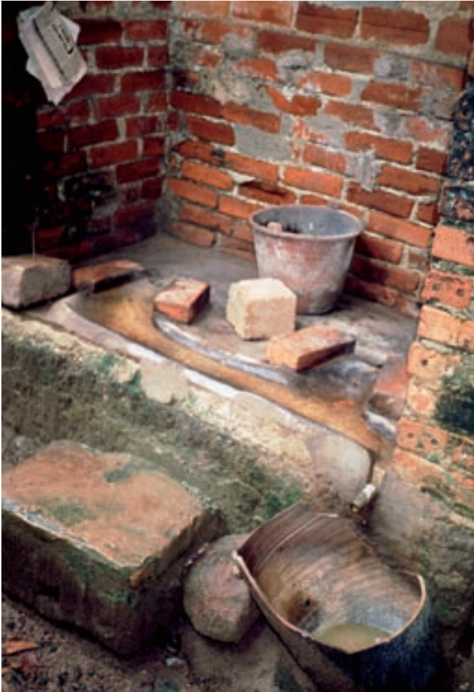
Double-pit latrine with urine diversion (Vietnam): latrine floor with openings to the two chambers for faeces, a urine diversion channel and a urine pot.
