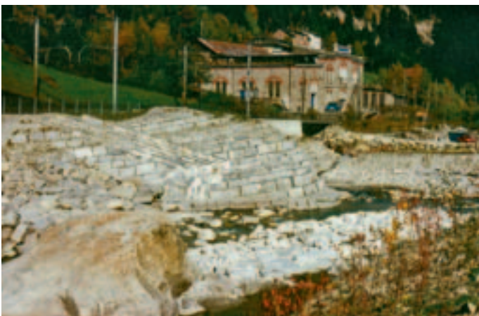
Fig. 3: Built-up bluff designed to stabilize meanders in Gurtellen-Wiler.
